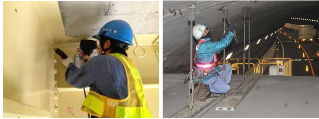
Fig. 1. Two inspection tasks: vision inspection and hammering test.
